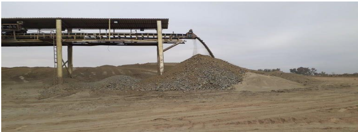
Figure 18 : zone de stockage
