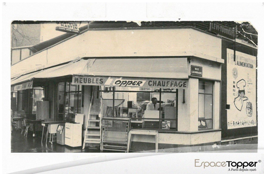
Figure N°31: the first TOPPER shop
